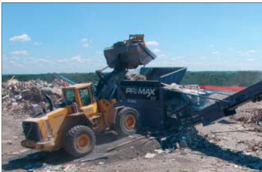
In the face of legal issues and declining landfill space, the Salem County Utilities Authority in New Jersey elected to recycle its landfill using primary reduction equipment.
