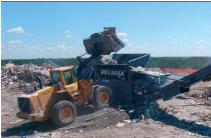
In the face of legal issues and declining landfill space, the Salem County Utilities Authority in New Jersey elected to recycle its landfill using primary reduction equipment.
